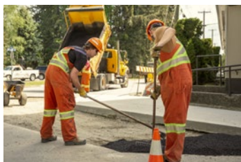
Neighbourhood roads, utility upgrades and lane paving
