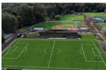
Start of construction on Gates Park soccer hub
