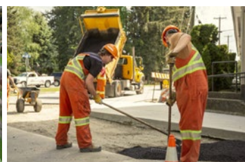
Neighbourhood road paving and utility upgrades
