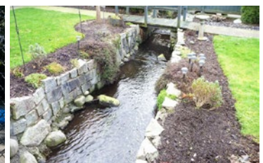
Upgrades to Maple Creek drainage
