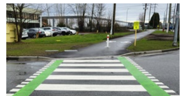
Kingsway Avenue improvements
