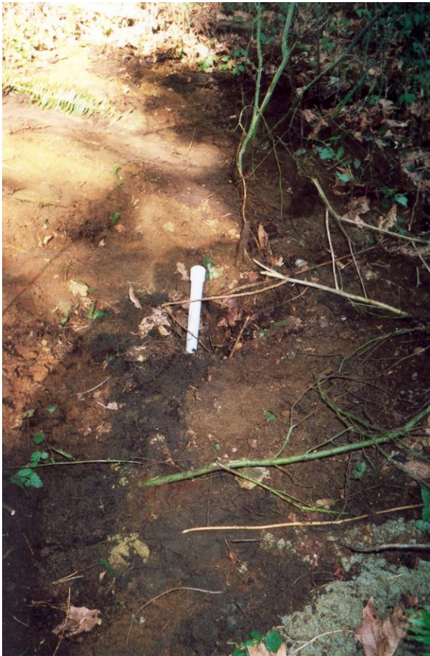
Photo 1. Completed standpipe piezometer installation at TH03-03.
