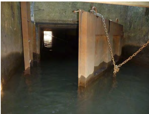
(a) Dyke Floodbox and Flapgate
