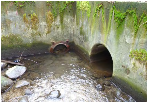
(a) 300 mm pipe to Maple is on left, 900 mm outfall from stormceptor & residential area on right.
