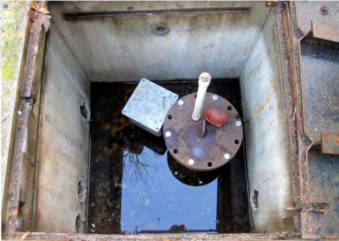
Photo 5. Surface completion of Maple Creek well.
