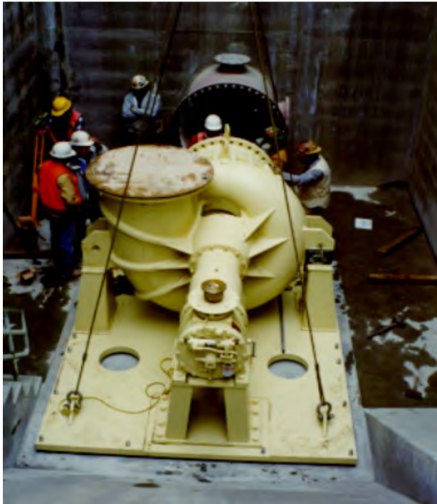
Photo 3-1: Dry Pit Hidrostral Pump (Red Bluff, California)
