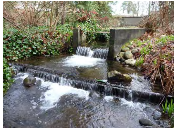
(b) Concrete Weir Downstream of Lougheed Hwy
