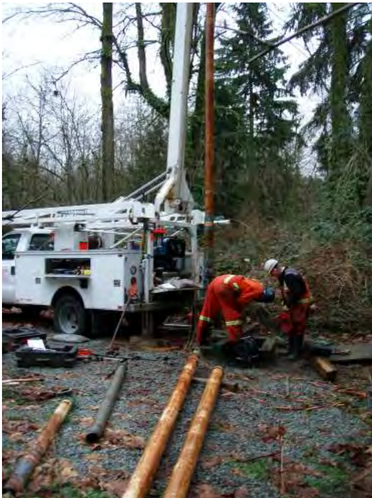
Photo 8. Pump and drop pipe pulled from Maple Creek well Feb. 16, 2011.
