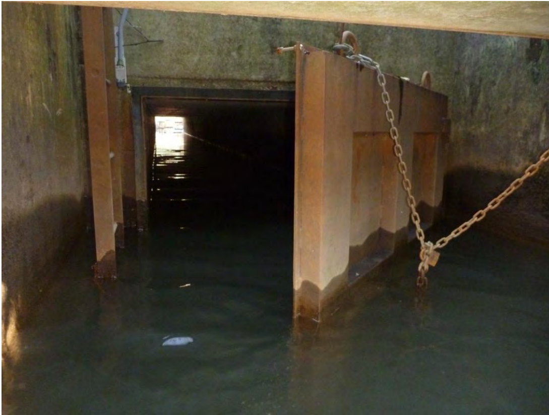
Photo 4-1: Existing Flapgate (with weight attached)
