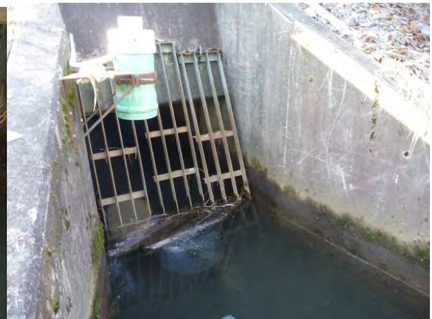
(b) Dyke Culvert Grill (upstream end)
