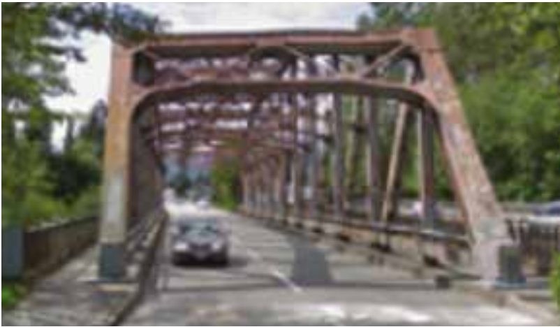
Eastbound Steel Truss Bridge
