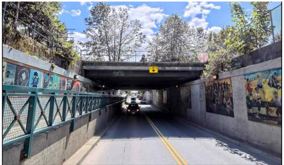
Shaughnessy Street Underpass (looking south)
