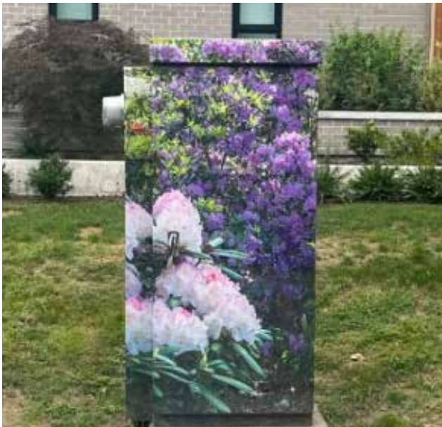
Utility Wraps in Port Coquitlam
