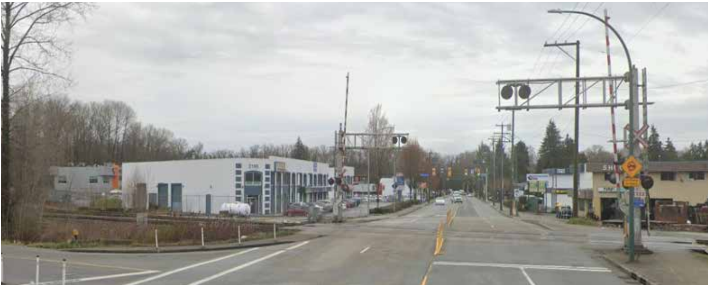
Westwood Street at Davies Avenue – Existing At-Grade Crossing
