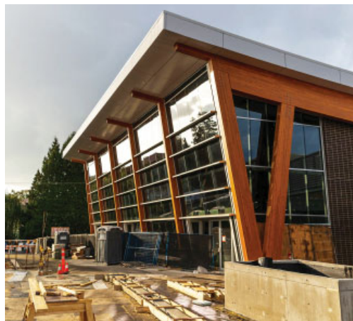
Investing in infrastructure
